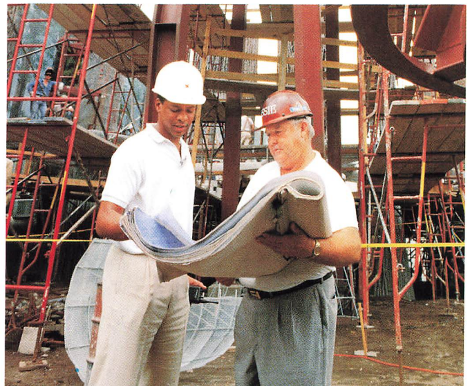
Construction crews build entrance to Star Tours at The Disney-MGM Studios Theme Park during summer. The attraction opens in January.
